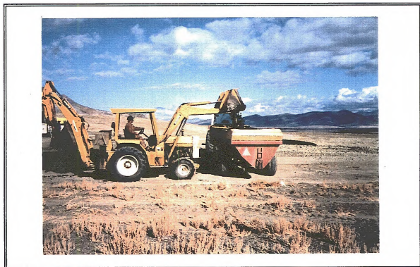
Photo 4: ARC donated backhoe/front end loader
